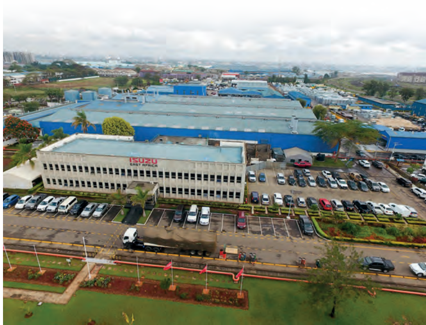
Aerial View of Isuzu EA Plant.
